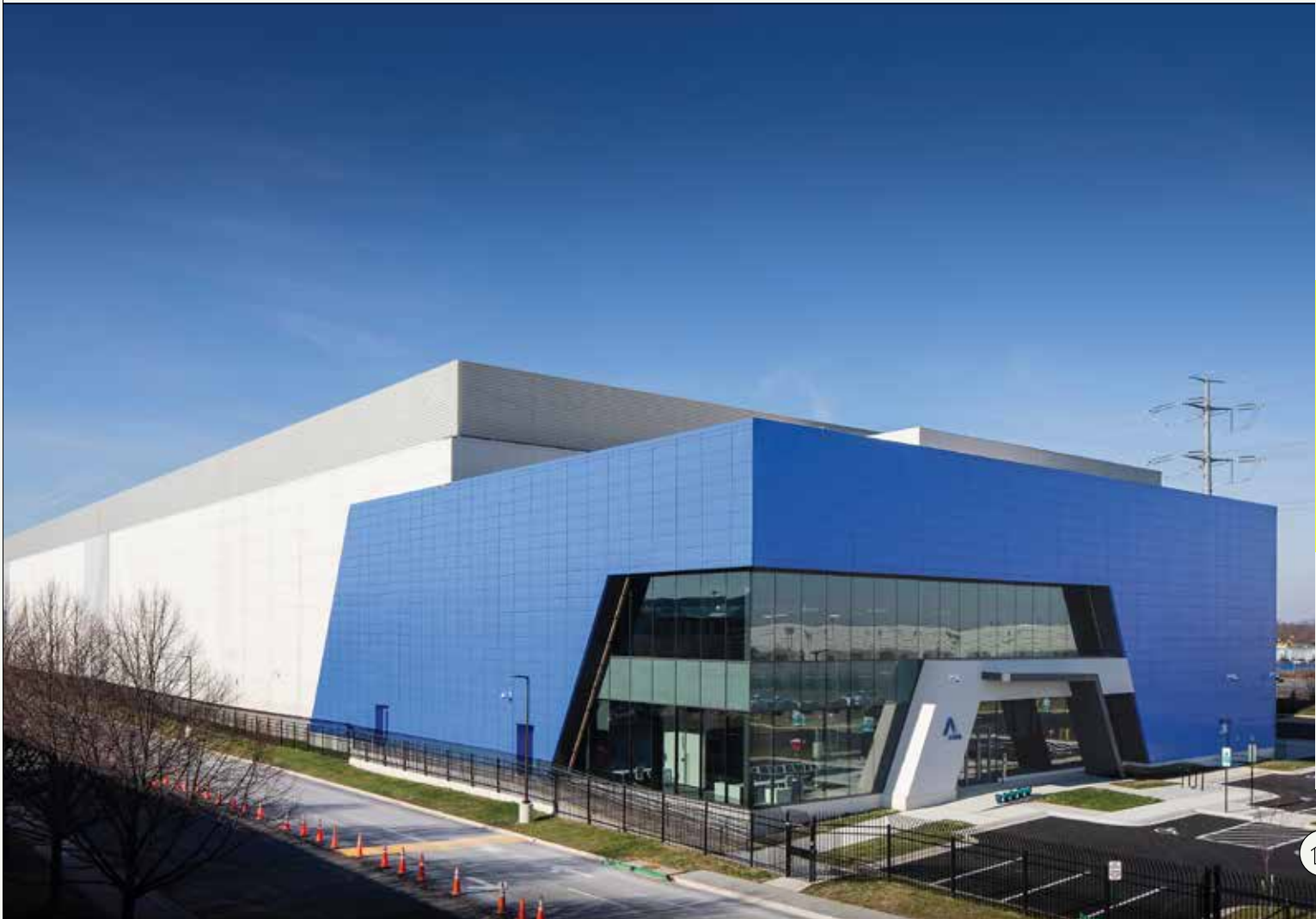
Aligned Data Centres use a closed loop air-cooled system that eliminates the need for water.
